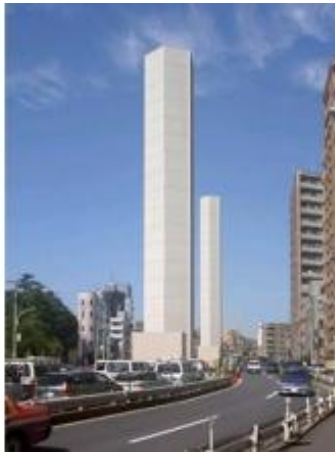
Figure 11. Exhaust stacks of the Central Circular Route
