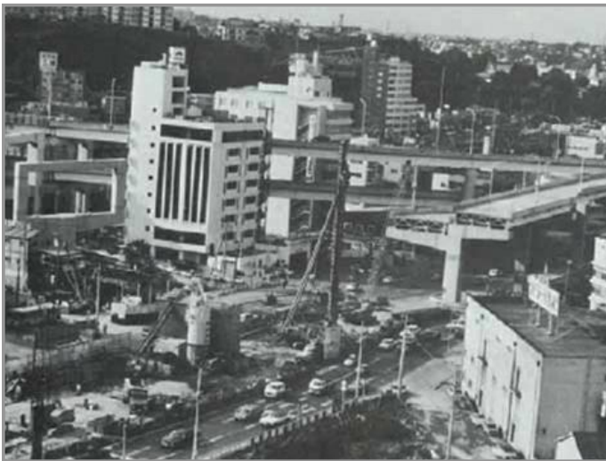
Fig 5. Highway construction in early stage in Tokyo
