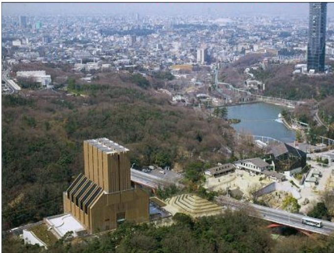
Fig 6. Ventilation station in metropolitan area
